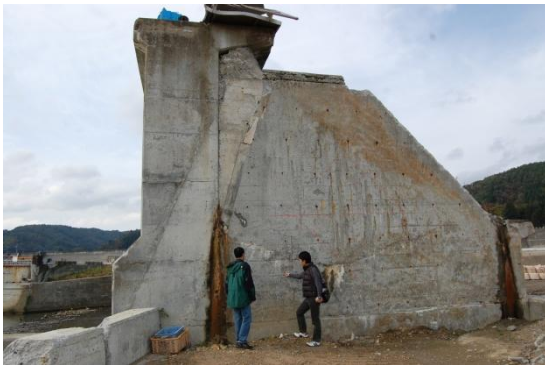
In the Taro district of Miyako City. An enormous embankment wall, which had been said to be “Best in the World,” was destroyed by the tsunami.
