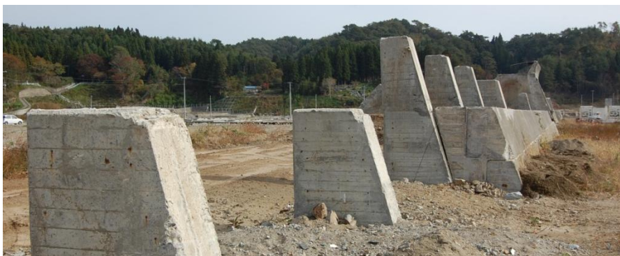
A 10 meter tall and 2.5km long sea wall called “The Best in the World.” The symbol of the Taro area of Miyako City, which was hailed as “The Tsunami Proof Town,” was destroyed by a 20 meter tsunami. Taken on the 30th of October, 2011.
