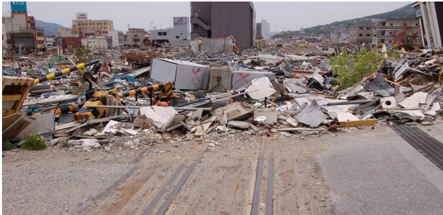
The center of Ofunato City with its destroyed railway lines. As of June 2012, neither the JR Ofunato line nor the Sanriku Railway minami-rias line have been repaired. Taken on the 19th of May, 2011.
