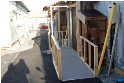
Temporary housing with wheelchair access in the Taro area of Miyako City.
