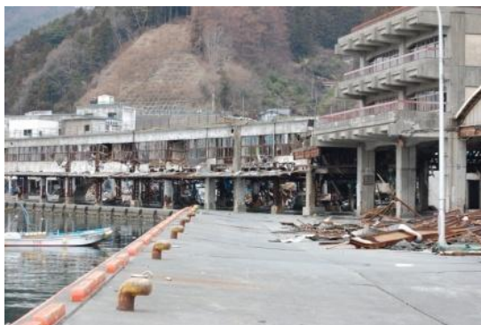
The harbor took a devastating amount of damage
